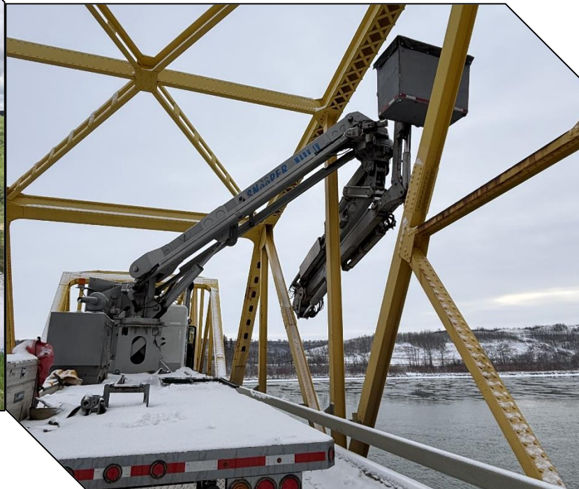
LEA PARK BRIDGE, AB
