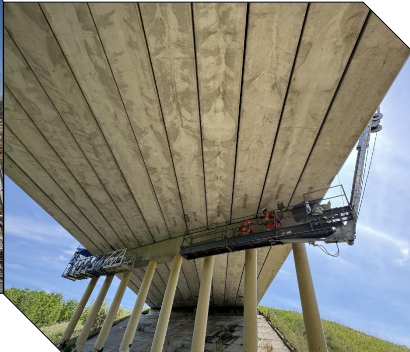
BITTERN LAKE BRIDGE, AB
